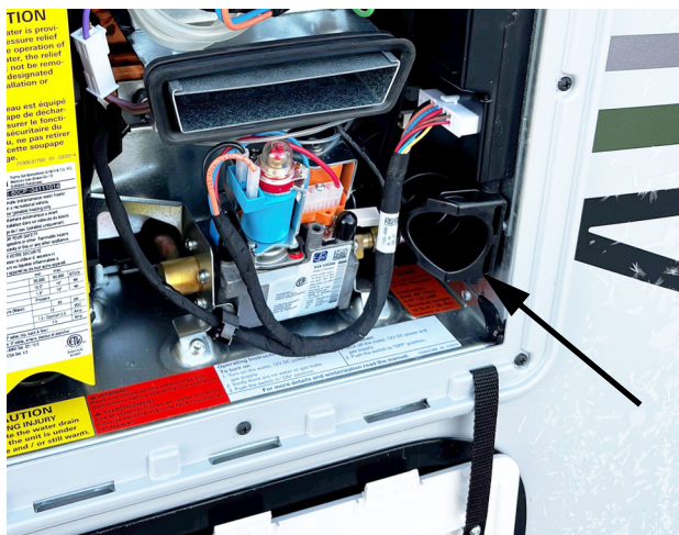
Water inlet strainer can easily be stored as shown above. -Typical View
