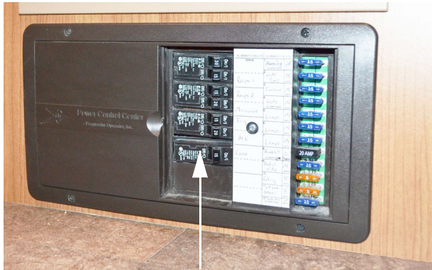
120-Volt Circuit Breakers -Typical View
