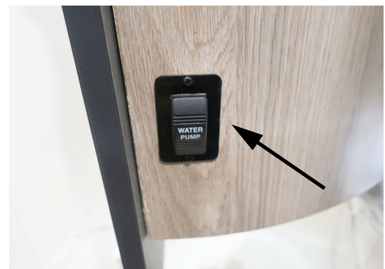
Water Pump Switch in the lavatory. -Typical View
